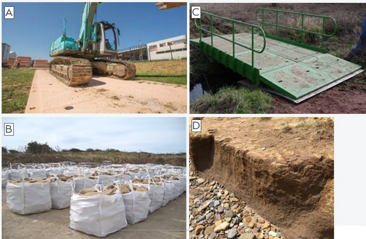
Figure 4.16: Sand bag and access track construction for temporary beach access
